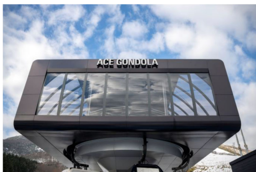
Ace Gondola mountain foot station building
