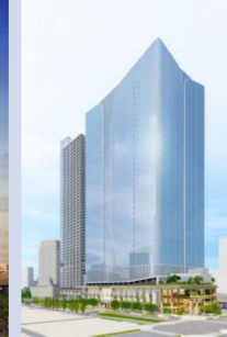
Nihonbashi 1-chome East Block Redevelopment Project Chuo-ku Commercial/Office/Conference, etc. Total floor space: 274 (A) Scheduled for completion in FY2031
