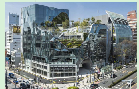
Tokyu Plaza Harajuku "Harakado" Shibuya-ku Commercial/Public facilities Total floor space : 20 Opened in April 2024
