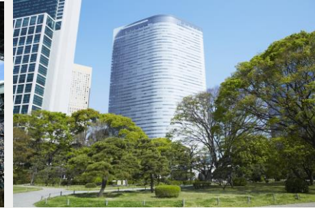
Dentsu Headquarters Building
