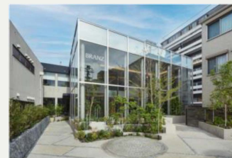
Building design that actively incorporates environmentally friendly materials
