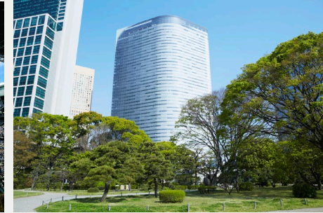
Dentsu Headquarters Building
