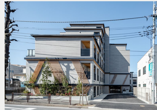
CAMPUS VILLAGE Ikuta (Completed in March 2024; total student condominiums units: 130) Tokyu Land Corporation has developed an environmentally friendly property: the first student residence with a large hybrid structure combining wood and RC construction.
