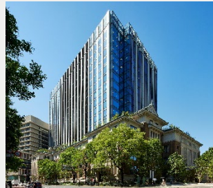
KUDAN-KAIKAN TERRACE Chiyoda-ku Office/Commercial Floor space : 68 Completed in July 2022
