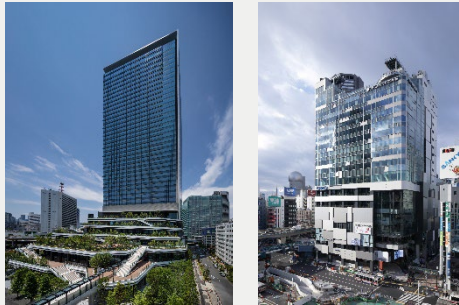
Major properties that have completed the switch to renewable energy (Left: Tokyo Port City Takeshiba, Right: Shibuya Fukuras)
