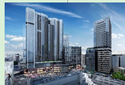
Shibuya Sakura Stage (Shibuya Sakuragaoka Block Redevelopment Plan) Shibuya-ku Office/Commercial/Housing Floor space : 255 Scheduled for completion in November 2023
