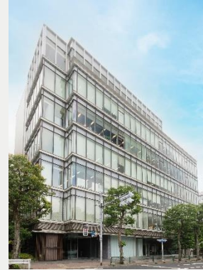
Meguro Tokyu Building
