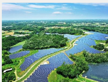
ReENE Namegata Solar Power Plant (Ibaraki) Rated capacity: 28MW (Operation started in FY2020)
