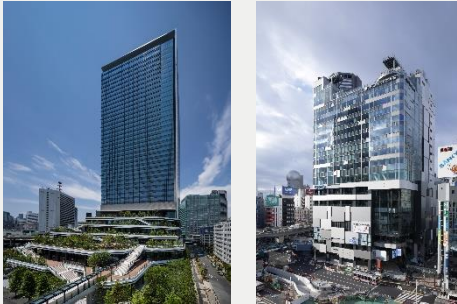
Major properties that have completed the switch to renewable energy (Left: Tokyo Port City Takeshiba, Right: Shibuya Fukuras)
