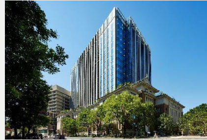
Newly constructed portion is cutting-edge office
