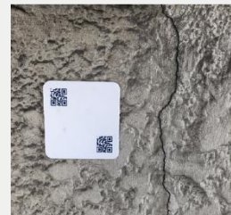
Capture inspection images
