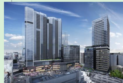
Shibuya Sakuragaoka Block Redevelopment Plan Shibuya-ku Office/Commercial/Housing Floor space : 255 Complete : November 2023 (Plan)
